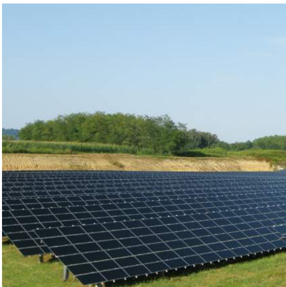
PV plant | San Giorgio (To - Italy)
