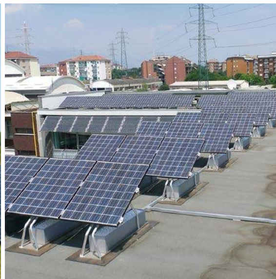
Roof mounted PV system | Rivoli (To - Italy)
