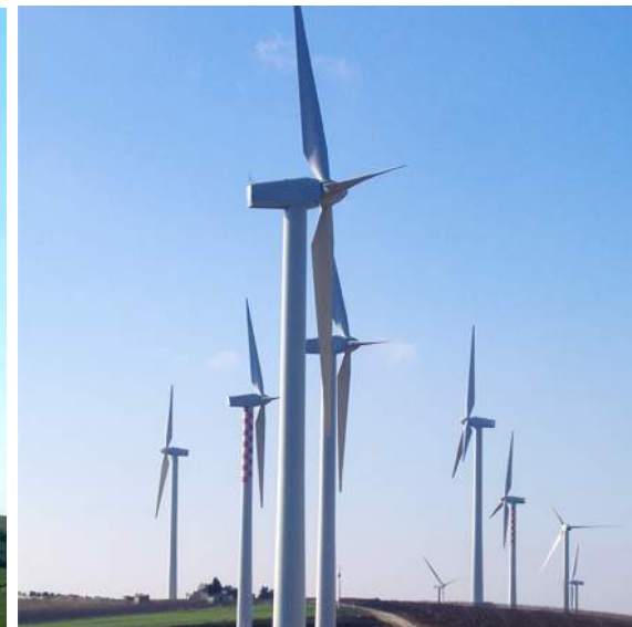
Wind farm | Fumosa (Tp, Italy)
