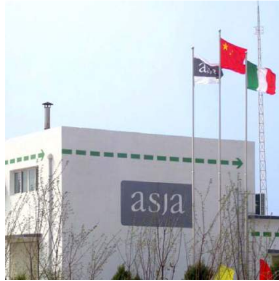
Landfill gas plant | Shenyang (China)
