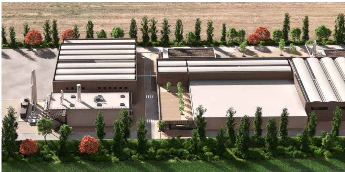
Biomethane production plant from OFMSW (Foligno, Pg - Italy)
